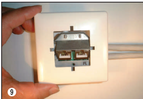
9. Place faceplate on socket. (each direction is allowed)
