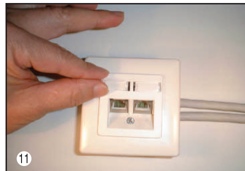
11. Place the ID label with plastic lens on frame.
