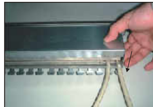
10. Push down the cover and snap into knob on each side.
