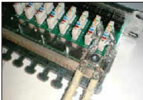
8. Complete the wires termination and cable mounting.
