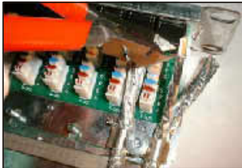
4. Cut each single wire's aluminum foil off subject to terminated IDC position length.
