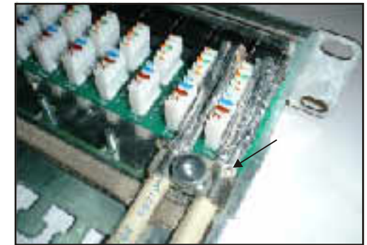
3-2. If STP cable OD<=6.0mm, bend back the copper braid and place braid under the bracket. Please place bracket exactly on the braid bending place.
