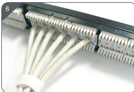
■ Use one velcro retaining strap to fix the six cables horizontally.
